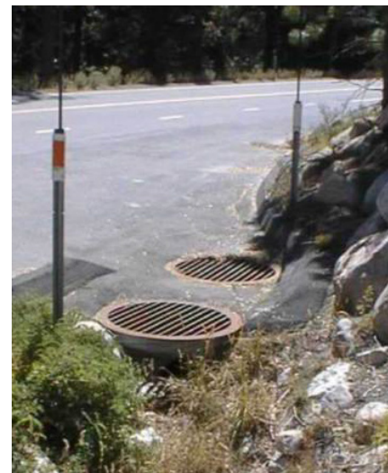
Caltrans Sand Can Sediment Trap (Double Barrel Modified CMP)
