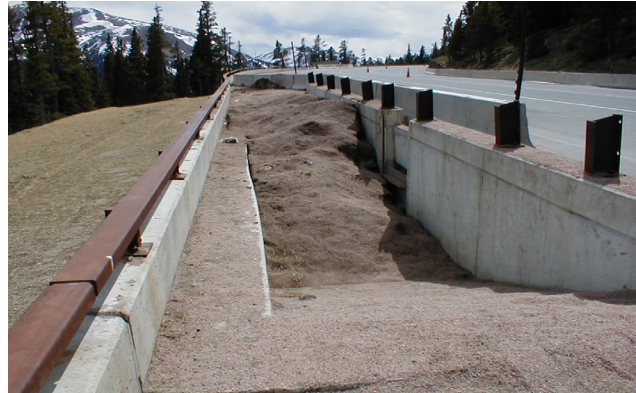
Berthoud Pass East Loading Dock Sediment Traps (not proposed for west side) (Source: CDOT)
