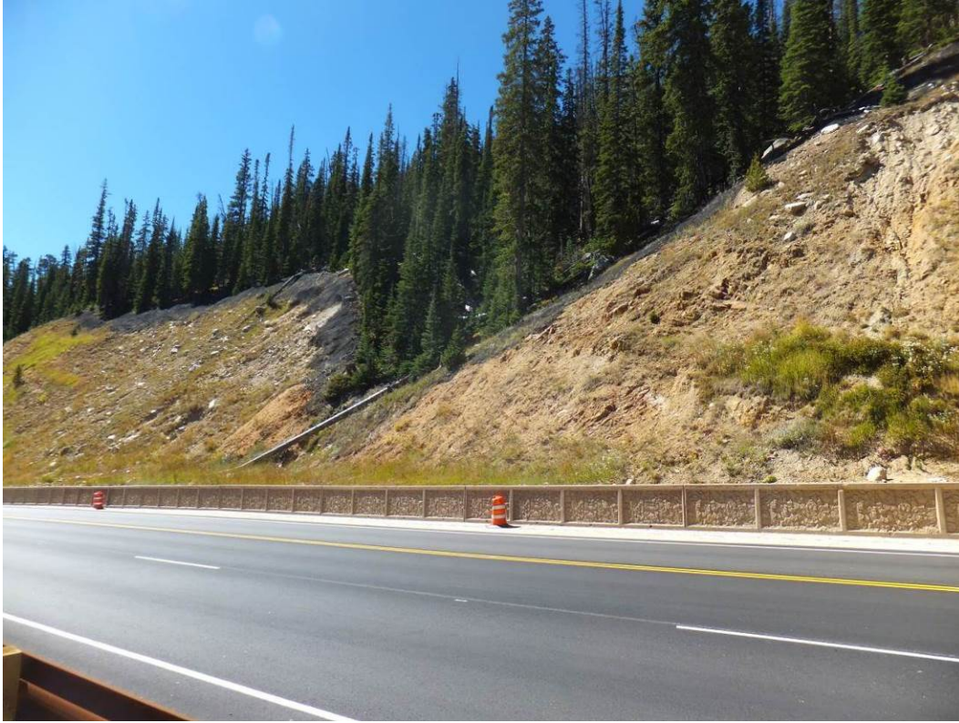
Figure 7-27. Milepost 237.38 (right) and milepost 237.35 (left)
