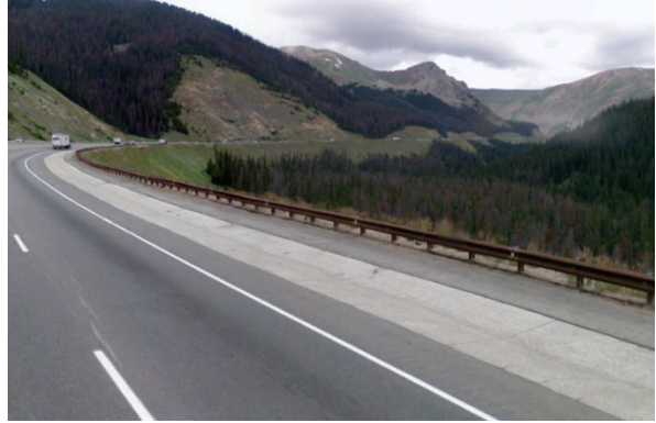
Valley Pan Drain west of Eisenhower Tunnel
