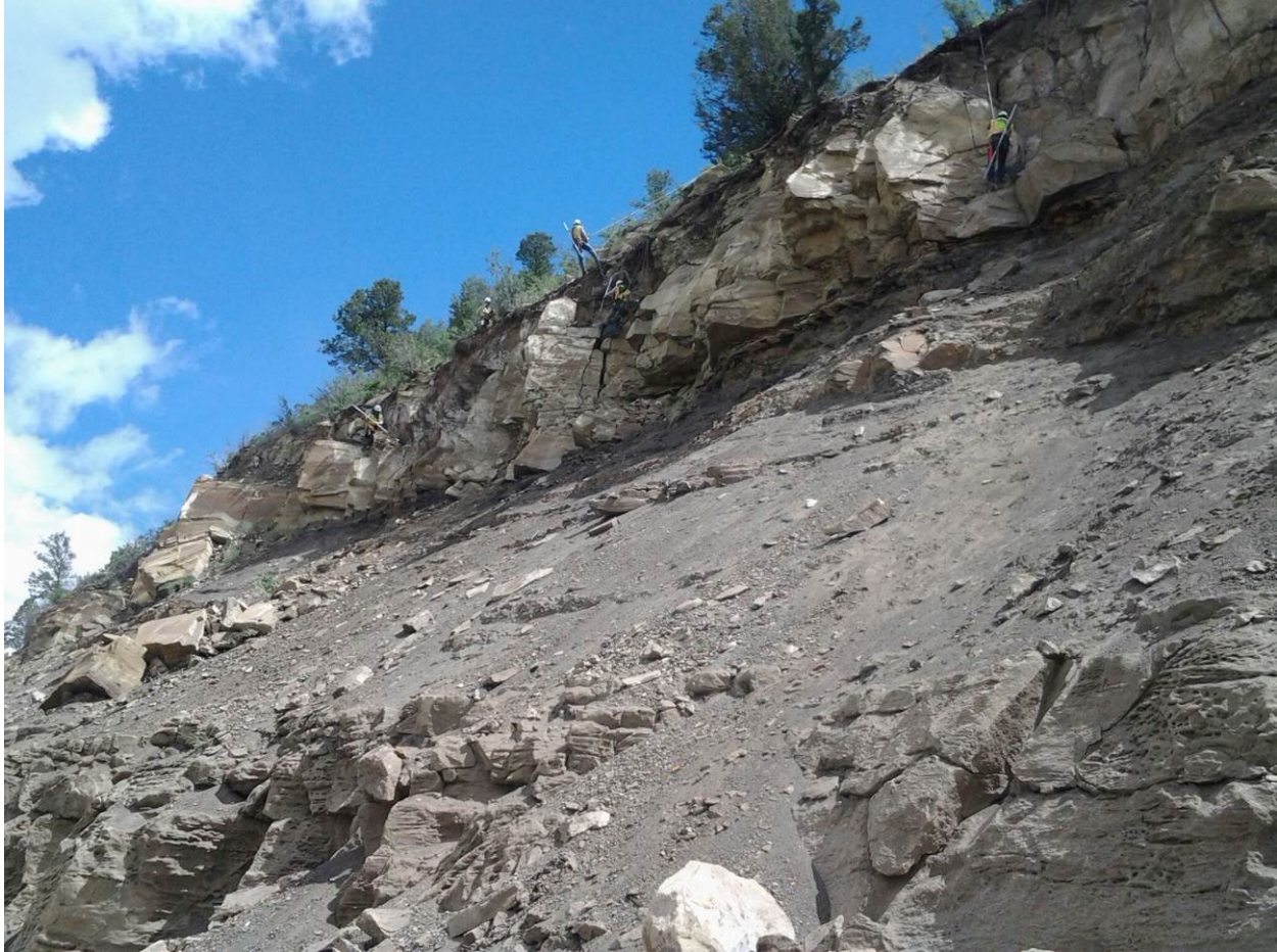
Figure 7-31. Manual scaling of a rock slope using scale bars
