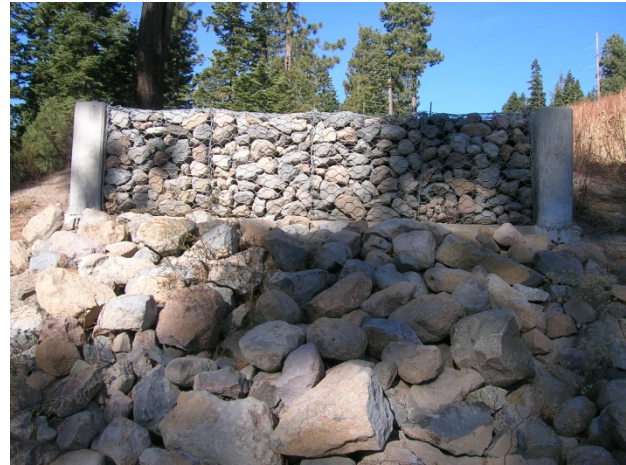
Downstream end of Caltrans Loading Dock Sediment Traps
