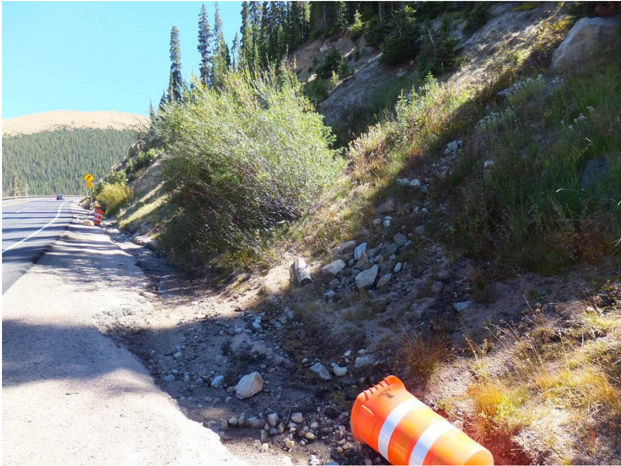
Figure 7-9. Naturally incised drainage ditch that serves as a catchment for small boulders between mileposts 241.28 and 241.3
