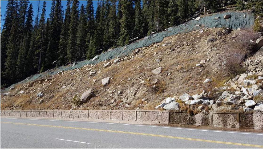
Figure 7-23. Milepost 237.6 A, slope of glacial till with erosion blanket at brow
