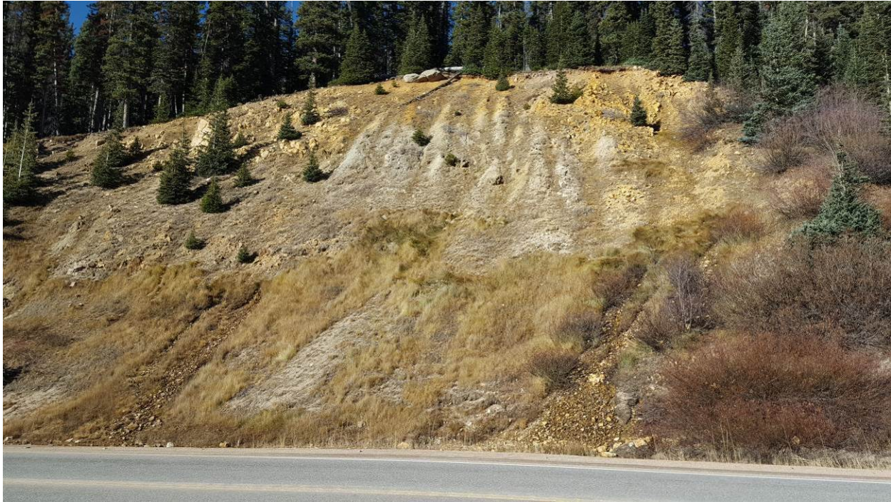
Figure 7-4. Milepost 241.95. The pocket of glacial till (gray) which was deposited in a channel or valley in the igneous bedrock (orange-brown)
