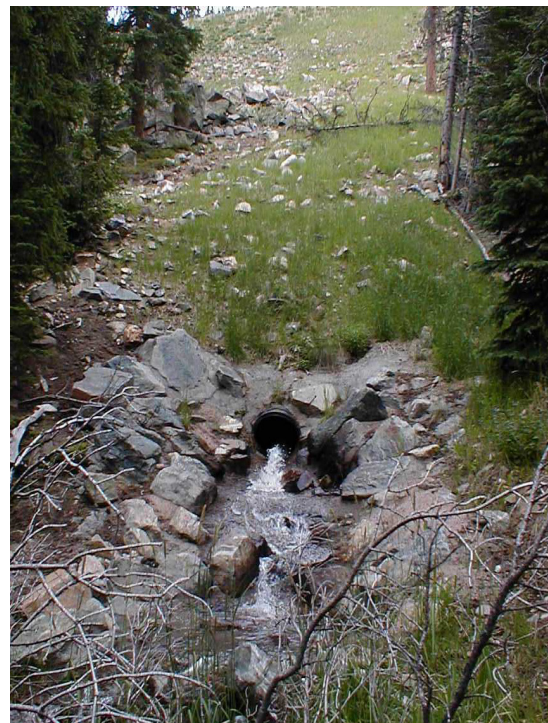
Buried Culvert Rundown with Riprap Outfall (Source: CDOT Straight Creek SCAP 2002)
