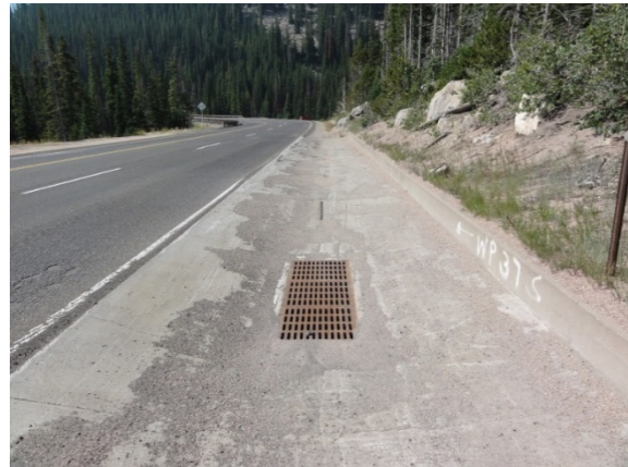
Valley Pan Drain west of Eisenhower Tunnel
