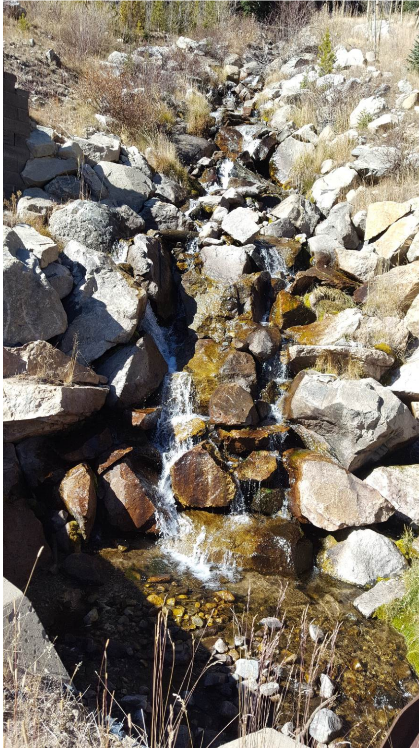
Figure 7-35. Example of an inlaid terraced rockery rundown feature at a tributary of Hoop Creek
