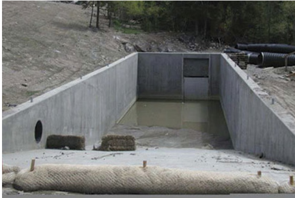
Berthoud Pass East Loading Dock Sediment Traps (not proposed for west side) (Source: CDOT)
