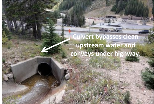
Clean Water Diversion at Loveland Ski Area Zip Creek Water Supply
