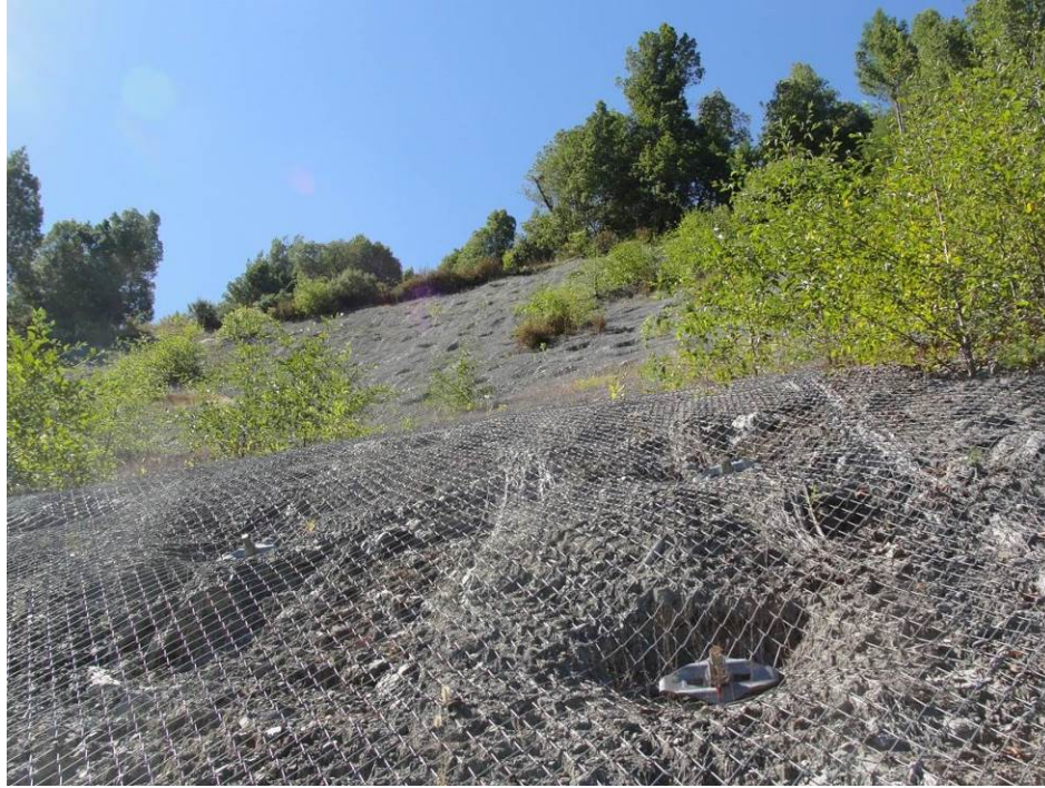
Figure 7-33. Example of pinned mesh
