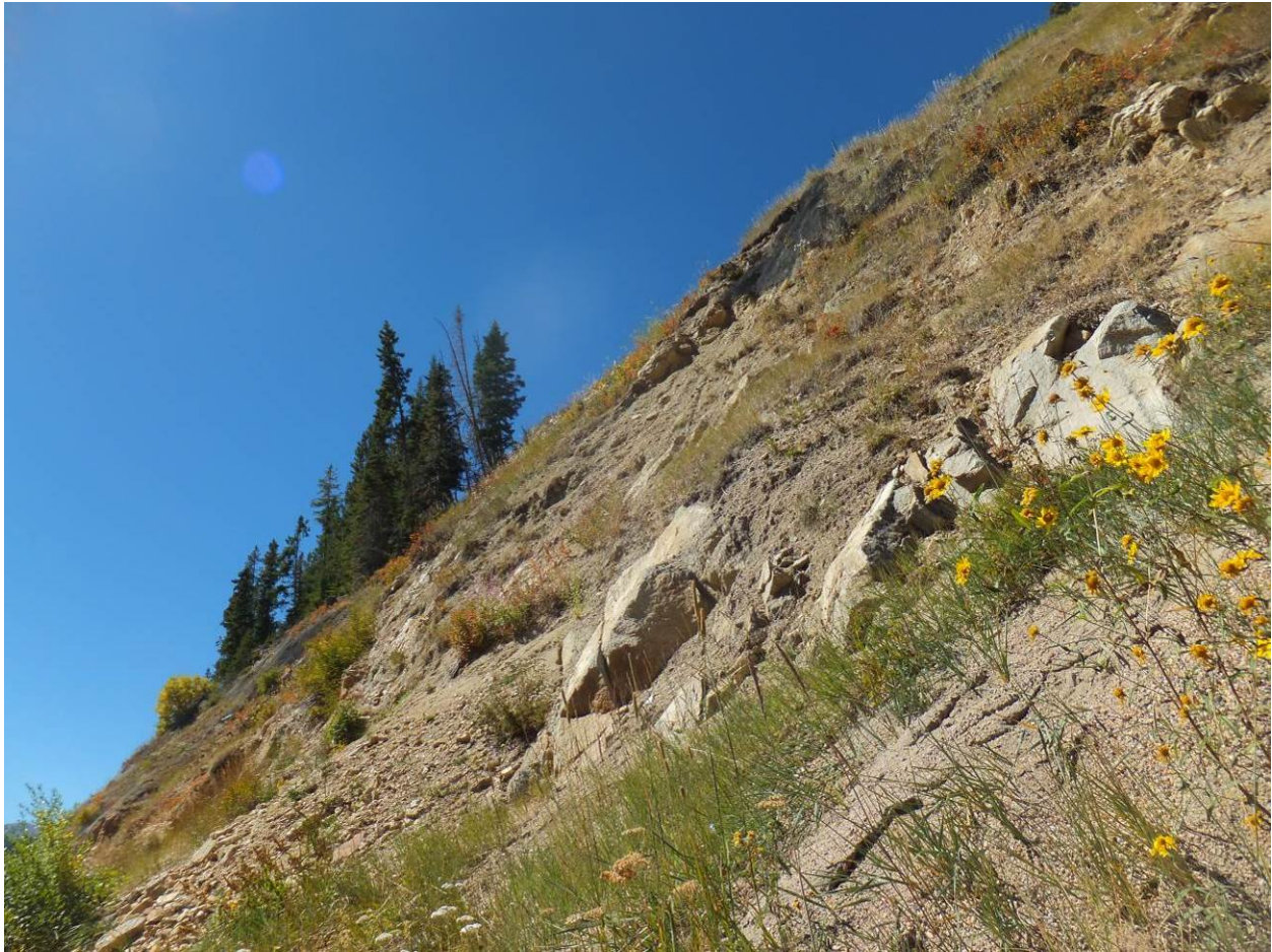
Figure 7-20. The upper slope at milepost 237.9, as viewed from the lower switchback
