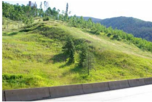
Figure 7-30. Photograph of revegetated slope (after rounding) from CDOT's Landscape Architecture Manual
