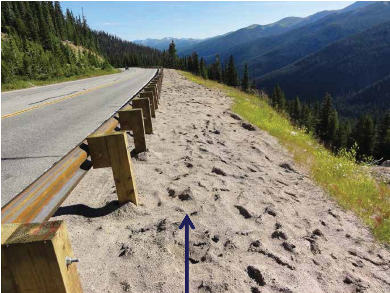
Graded bench to capture sediment
