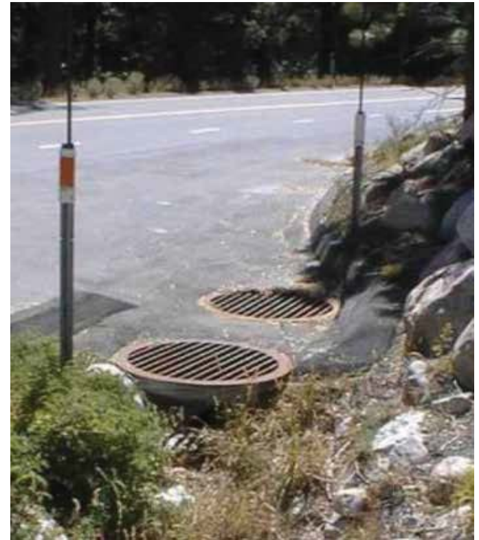
Inlet Traps or "Sand Cans" - Double Barrel Modified CMPs
