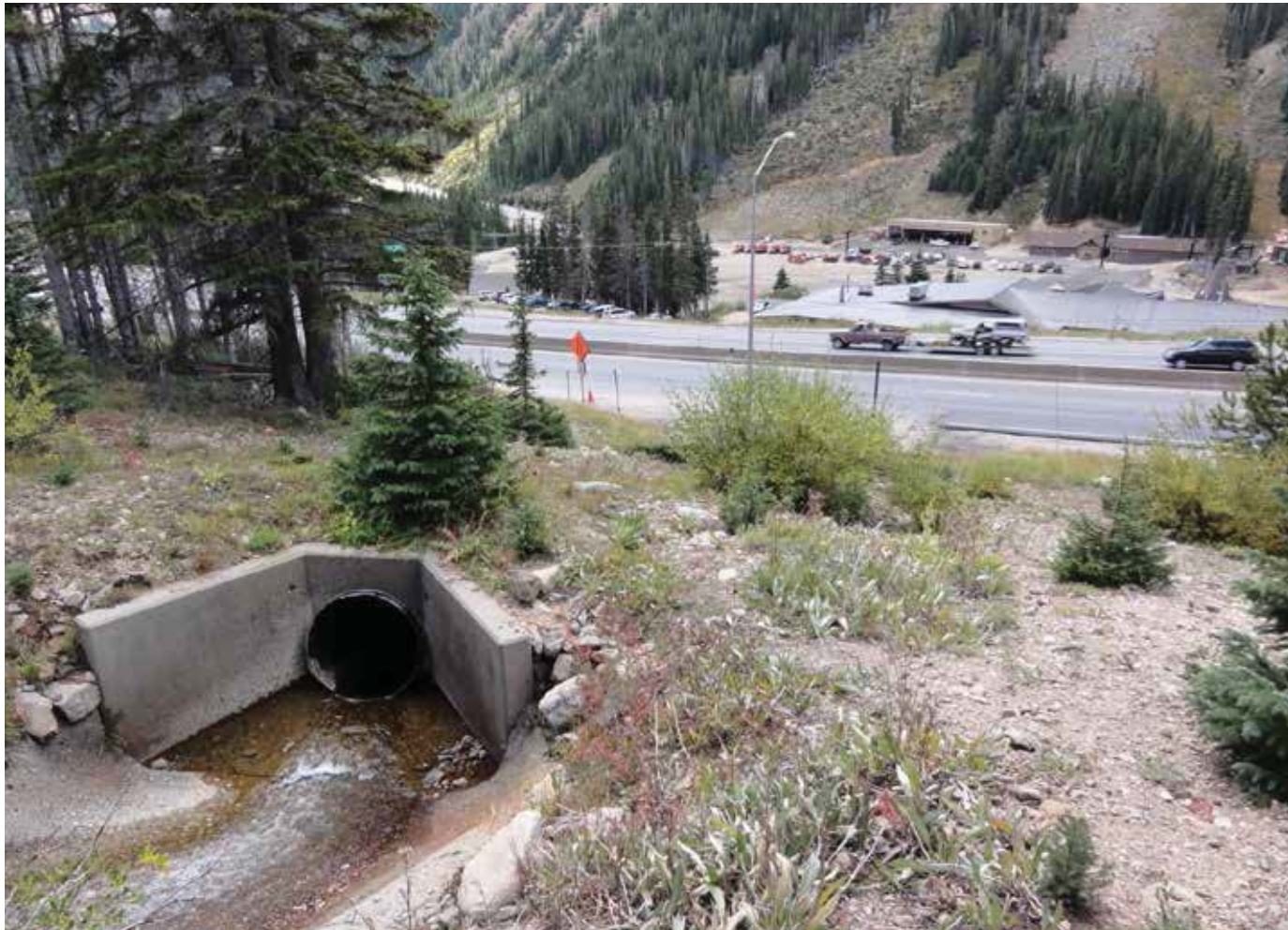
Culvert bypasses clean tributary water under highway
