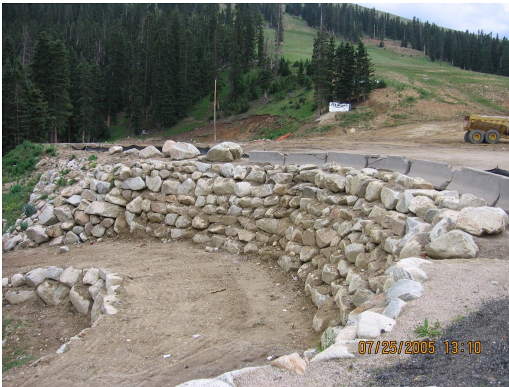
Figure 2. View of retaining wall and access road, just after construction, July 2005.
