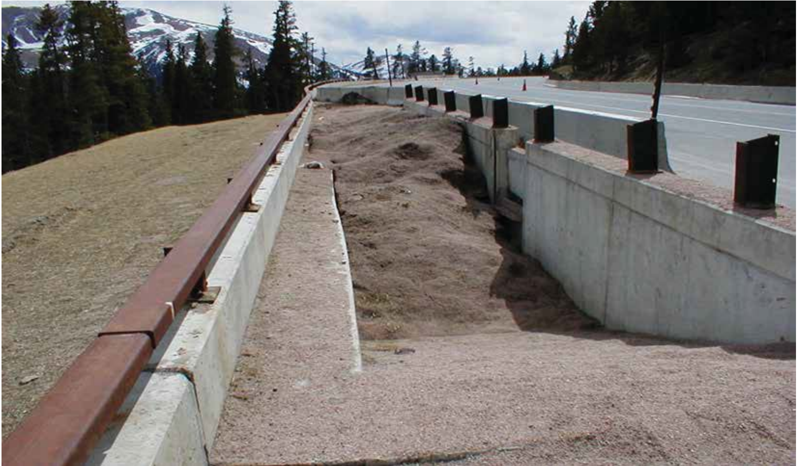
Berthoud Pass Sediment Trap
