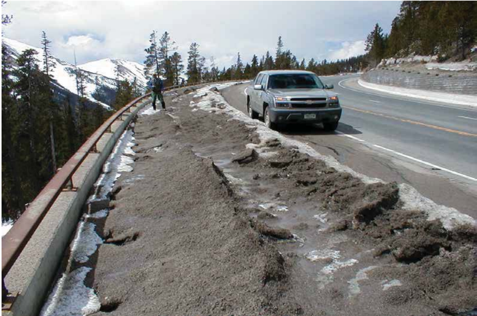
Sediment accumulation in snow storage area on Berthoud Pass
