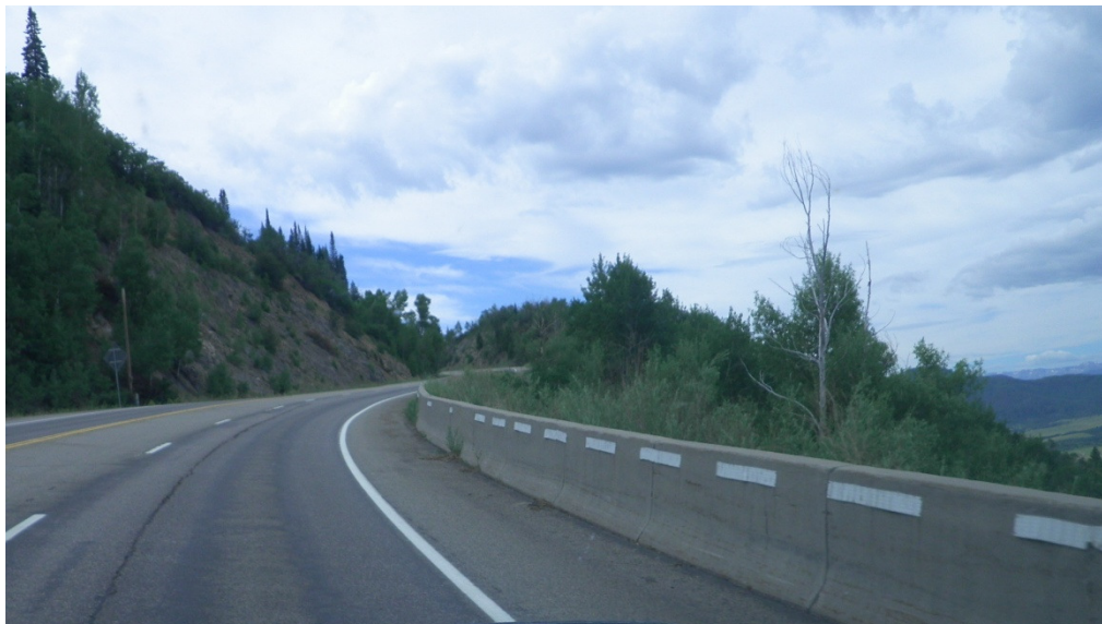
Jersey barrier in use on the west side of Rabbit Ears Pass.
