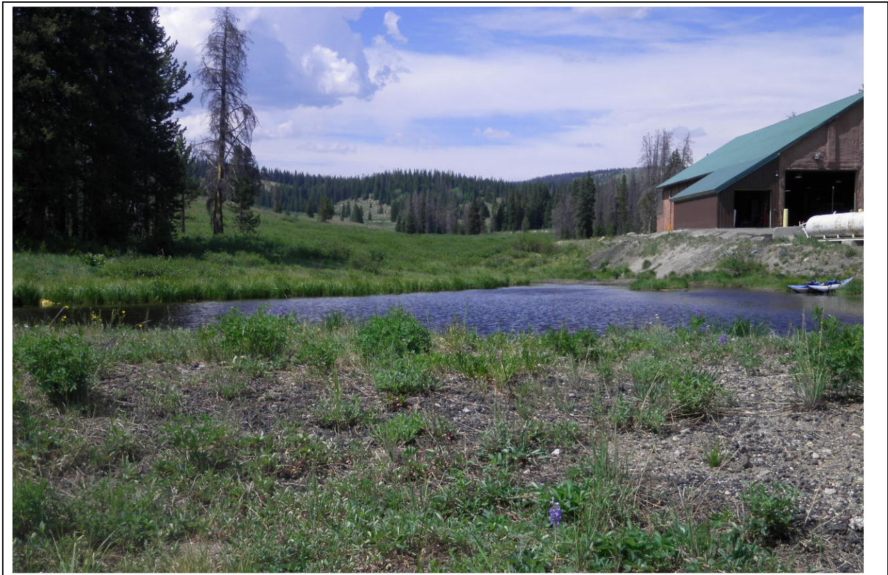
Figure 14. View looking north across the pond at the CDOT maintenance shed.
